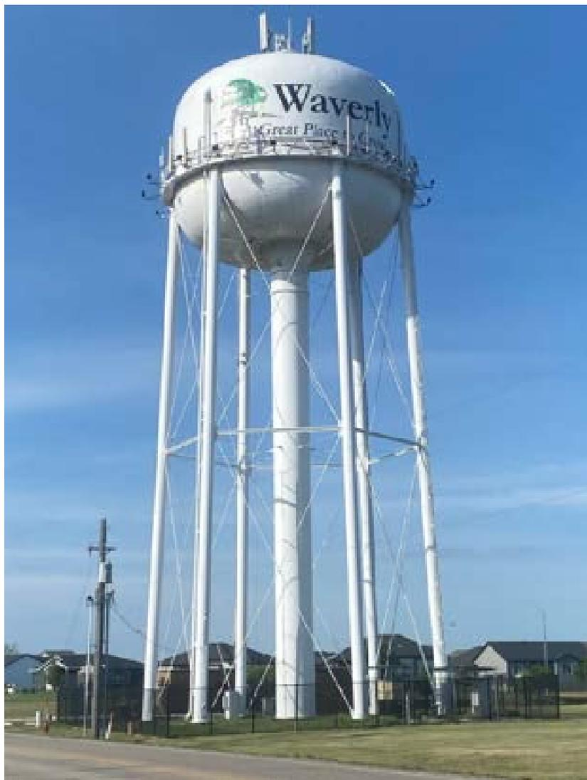
Figure 7. 500,000-Gallon Elevated Water Tower
